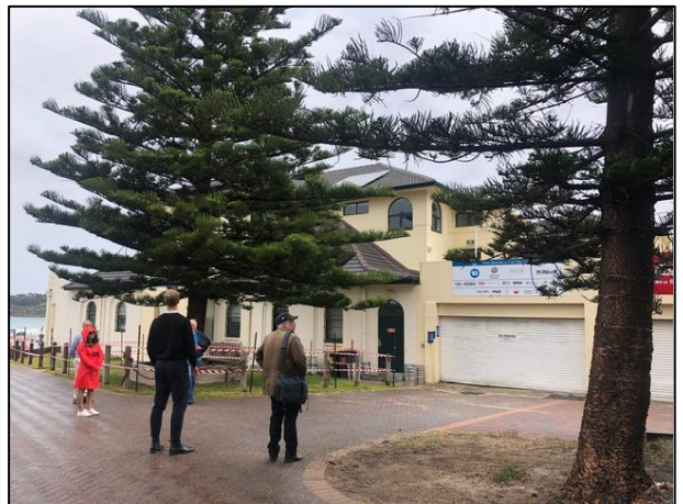
Figure 2: Club viewed from the north-east within Bondi Park
